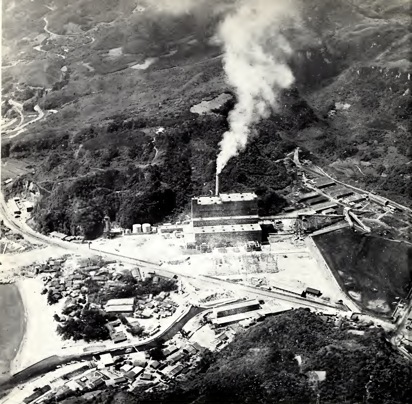
EXPANDING TO MEET DEMAND: the generating capacity of the Shenao Thermal power plant was doubled to reach 250,000 kw. in a major development project completed during 1966.
